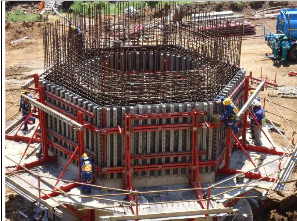
Base of inlet tower under construction.
