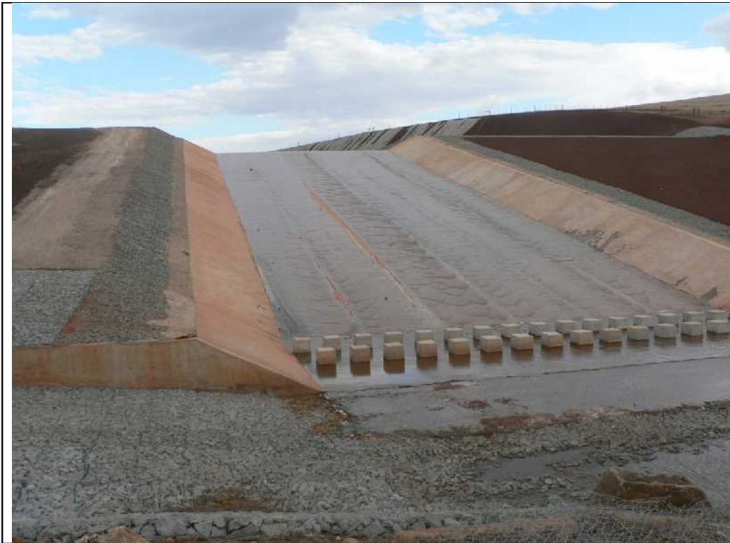
Cengane Dam, Owner: OR Tambo District Municipality
