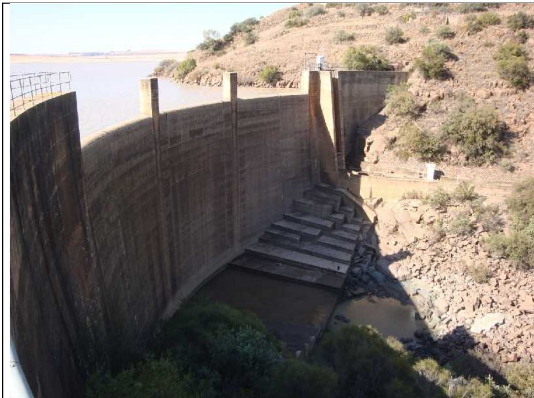
Downstream view of the Egmont Dam from the right bank.
