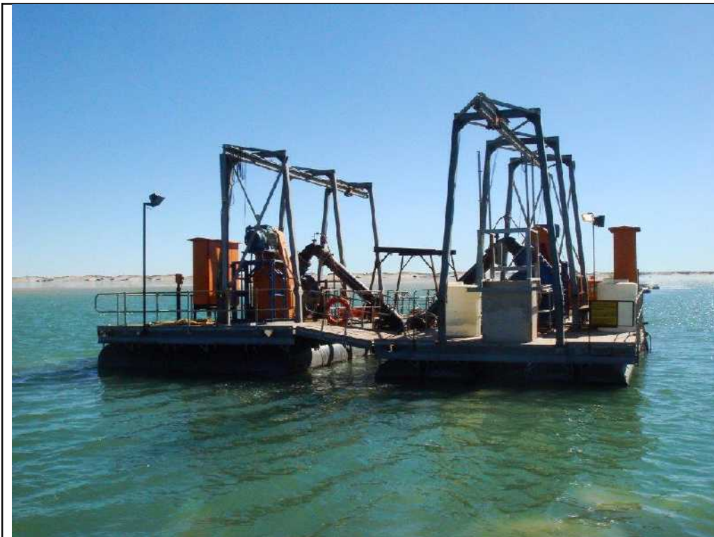
Kareerand Tailings Dam
