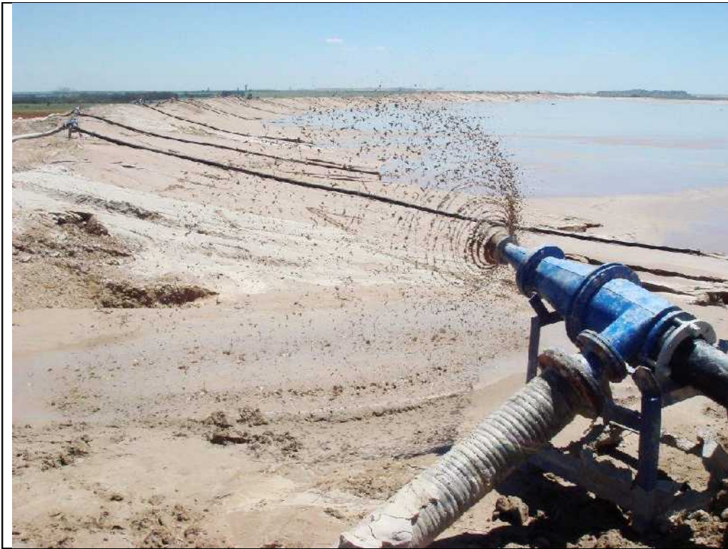
Kareerand Tailings Dam in the operational phase
