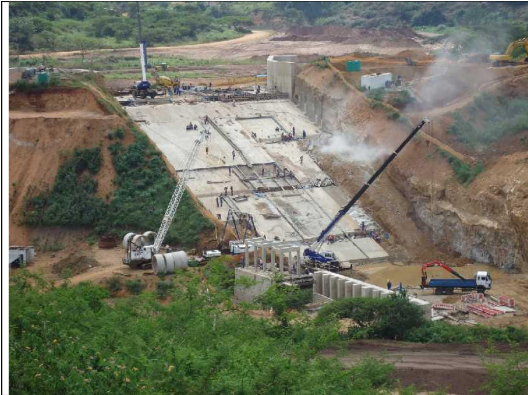
View on spillway.
