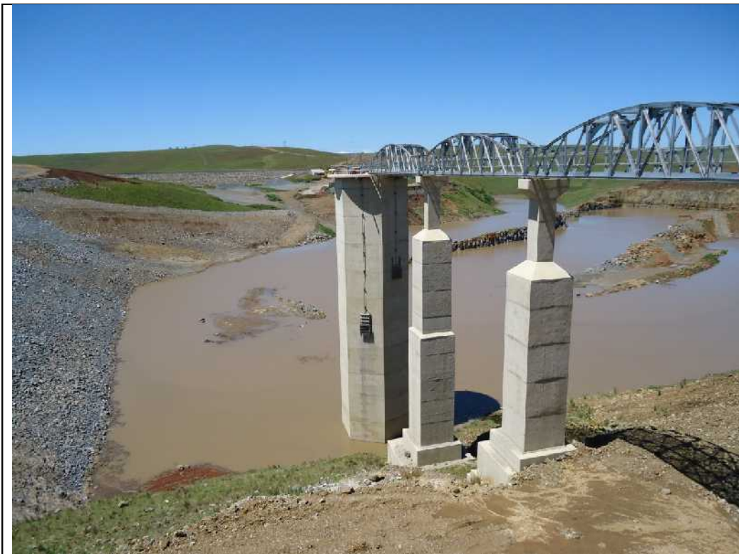
View of intake tower and access bridge.
