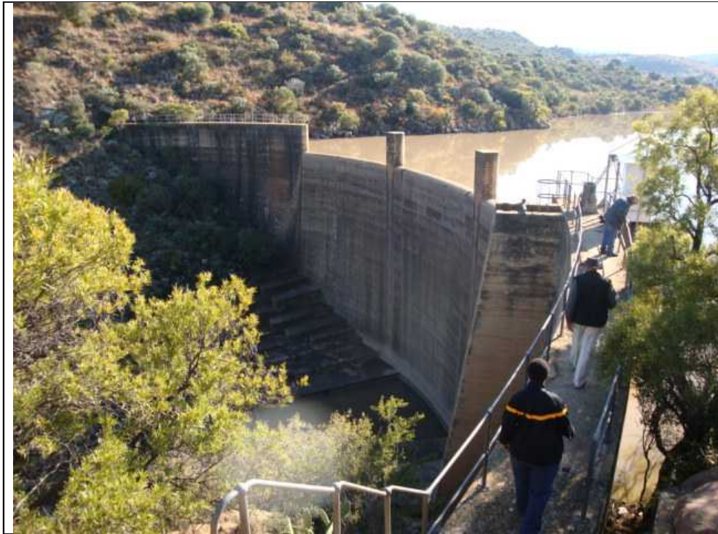
Downstream view of the 25m high Egmont Arch Dam near Wepener in the Free State from the left bank.
