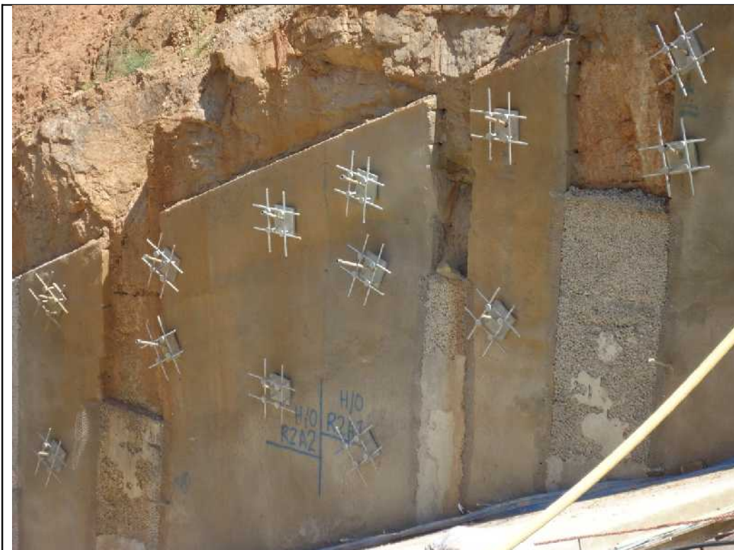
Picture shows soil nails and drains underneath spillway lining.
